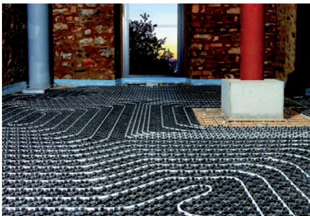
Fig. 72: Embedded heating/cooling provides cosiness and comfort also in old buildings
