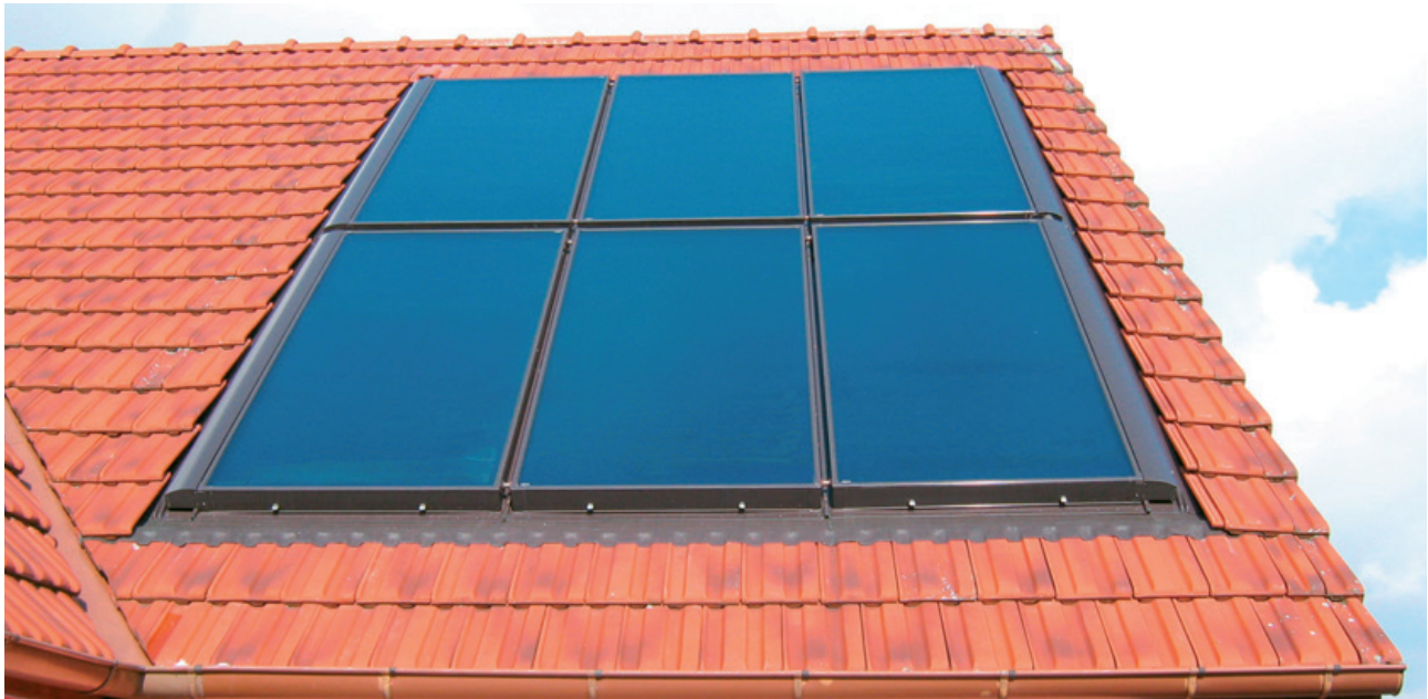
Fig. 56: Example of flat plate collector installations
