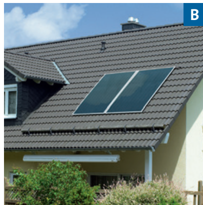
Solar thermal system for domestic hot water
