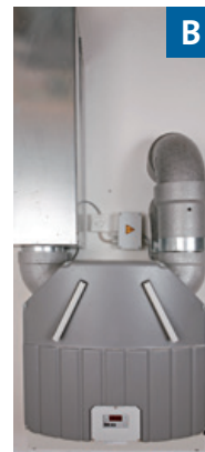
B Controlled apartment ventilation with heat recovery
